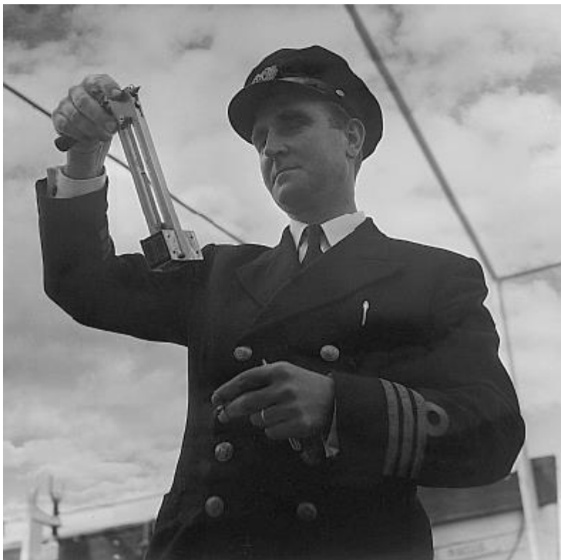
observer reading sling psychrometer (photo KNMI, circa 1960)
